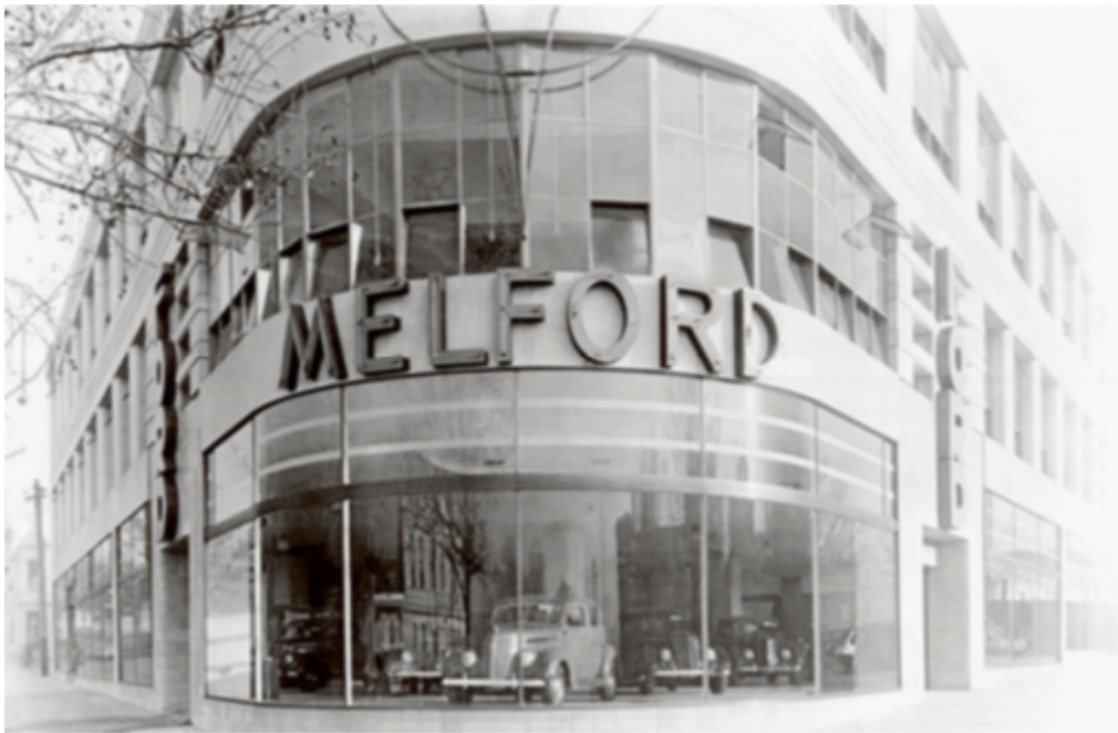
Figure 8. "On the Fringe of a Business District." Melford Motors, Elizabeth Street, Melbourne, Harry A. Norris, 1937. Construction and Real Estate Journal, 24 November, 1937, p.7.
