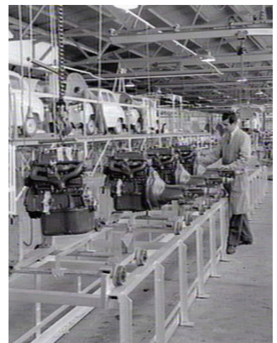
Austin Assembly Line, Melbourne, 1956, SLV H92.20/5803.
