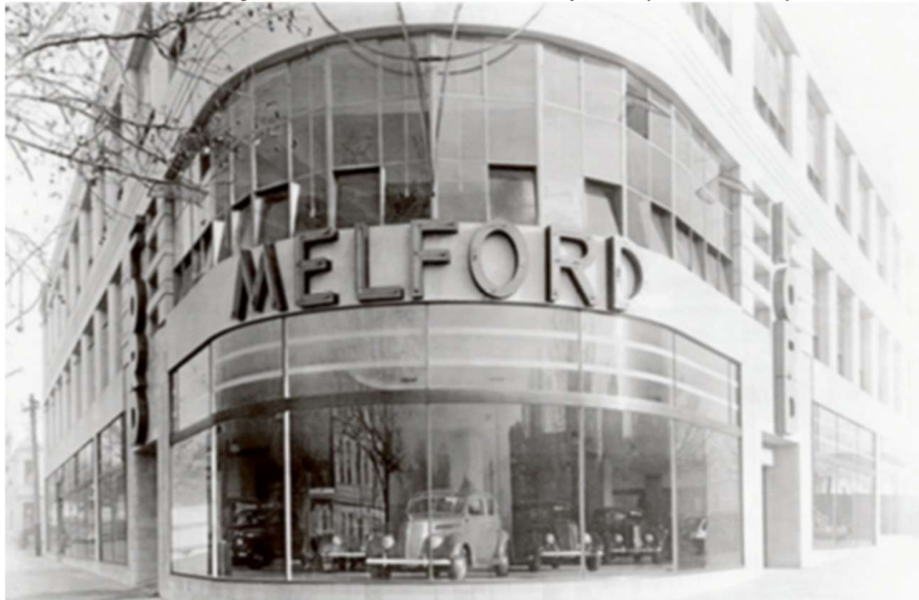
Figure 8. "On the Fringe of a Business District." Melford Motors, Elizabeth Street, Melbourne, Harry A. Norris, 1937. Construction and Real Estate Journal , 24 November, 1937, p.7.
